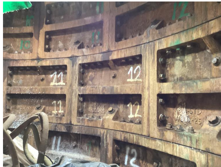
Conditions Post-Liner Grouting
