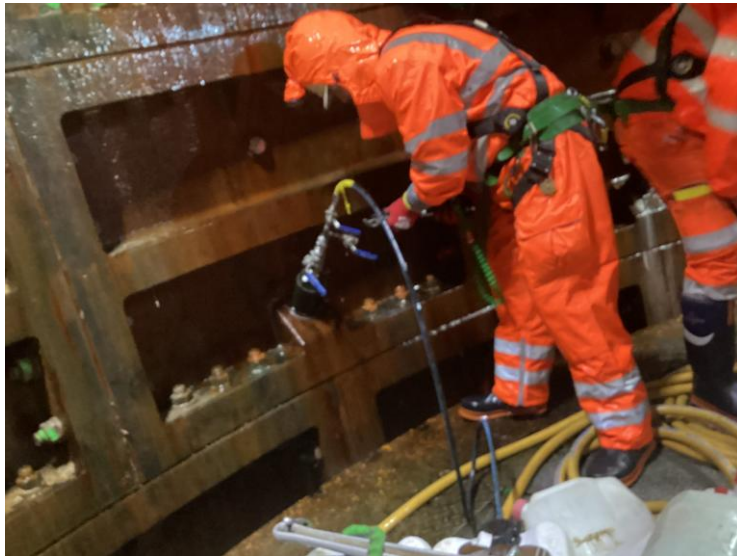
Conditions Pre-Liner Grouting
