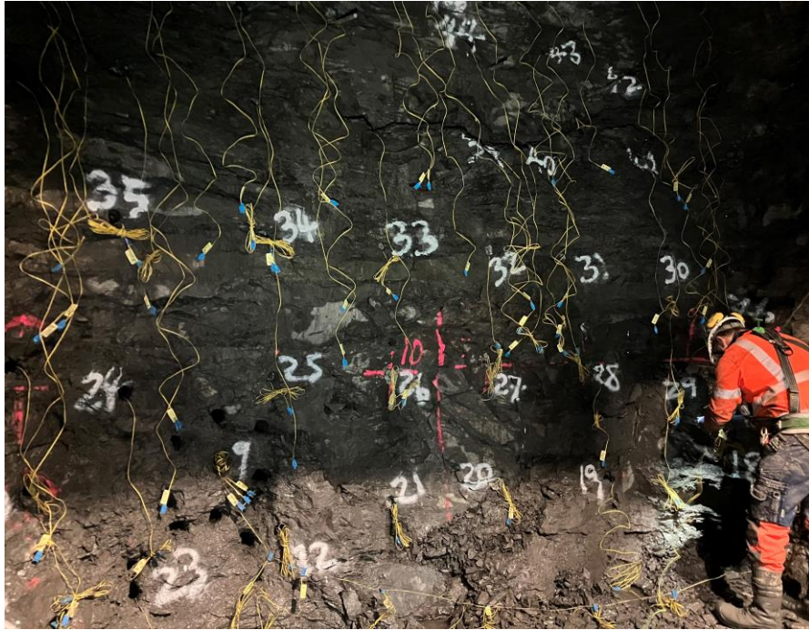
The cubby face charged in preparation for the second blast within the Production Shaft
