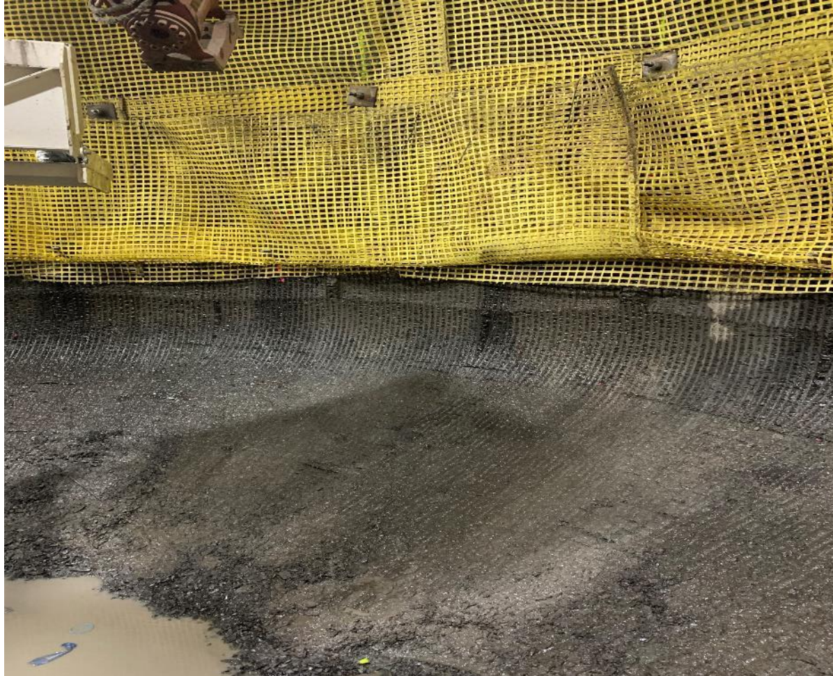
Ground support from the bench using hand borers and air legs
